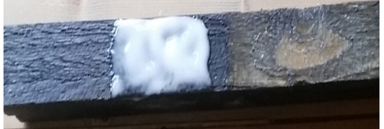
Painted wood surface • Paint Remover applied • Wiped off and paint removed
